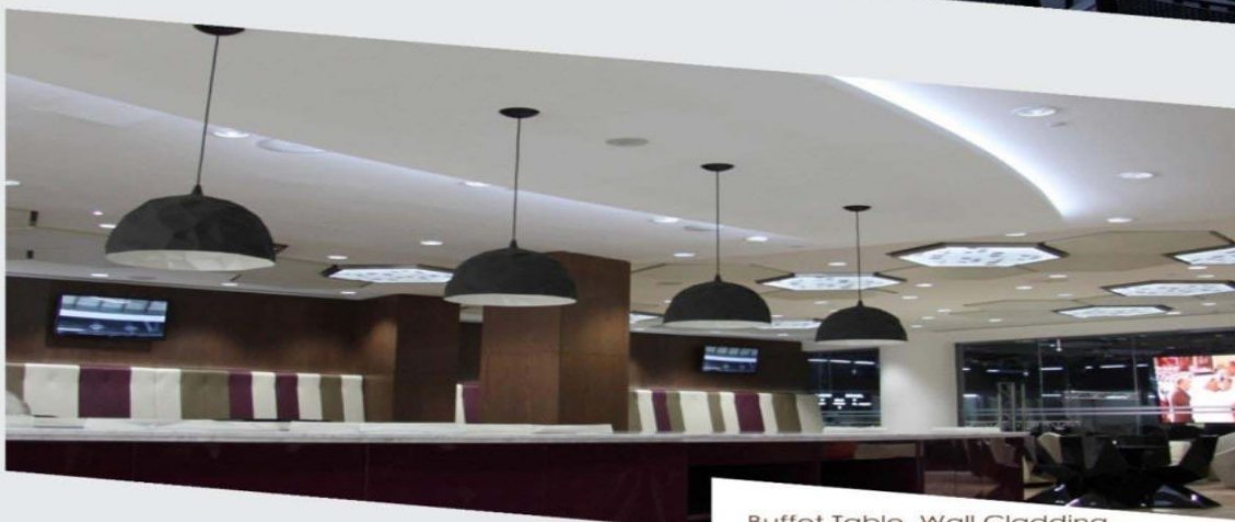
Buffet Table, Wall Cladding , Ceiling Hexagon Panels from stainless steel and acrylic sheets
