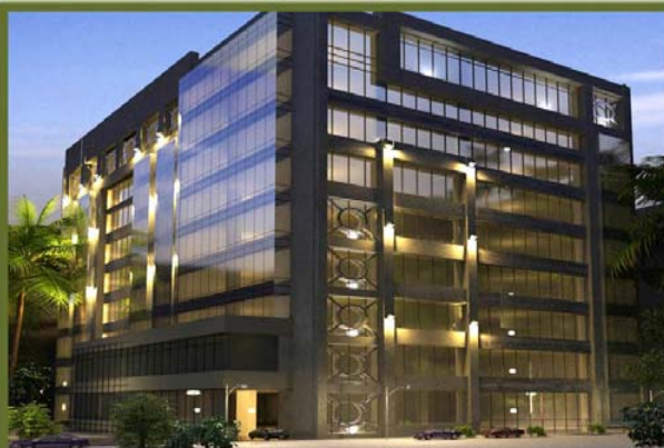
COMMERCIAL & OFFICE BUILDING (3B+G+M+7TY) AT BIN MAHMOUD
