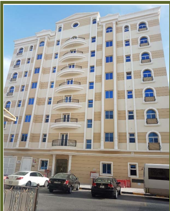
RESIDENTIAL BUILDING (2B+G+7) AT MUNTAZAH
