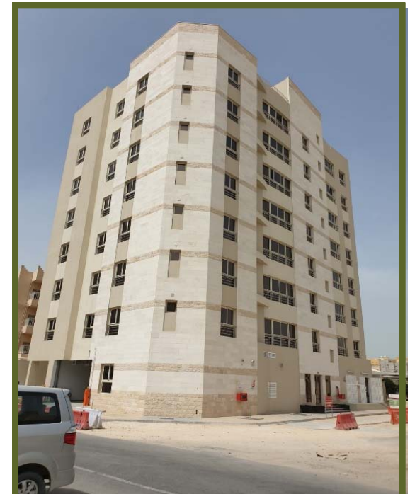
RESIDENTIAL BUILDING (B+G+7) AT AL SADD (140)
