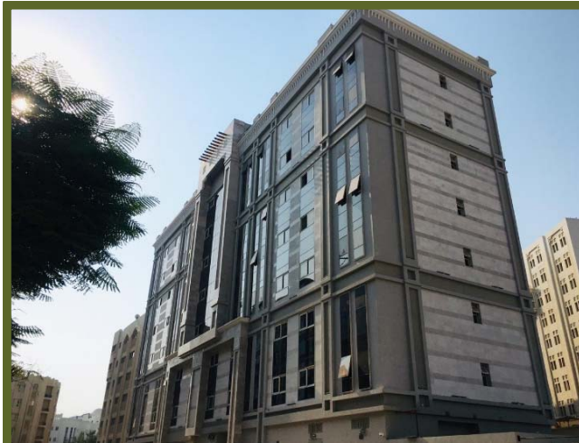
(2) RESIDENTIAL BUILDING (B+G+7) AT BIN MAHMOUD (155)
