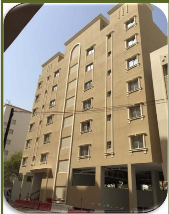
RESIDENTIAL BUILDING (B+G+6) 18 FLAT AT NAJMA
